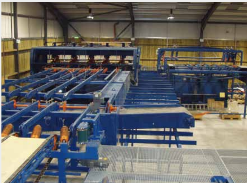
Assembly of the primary stacking line in the Irish company ECC. The secondary stacking line can be seen on the right.
