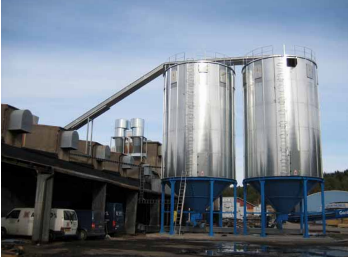
The fully automated briquetting plant can handle several thousand kilos of woodchip per hour.
